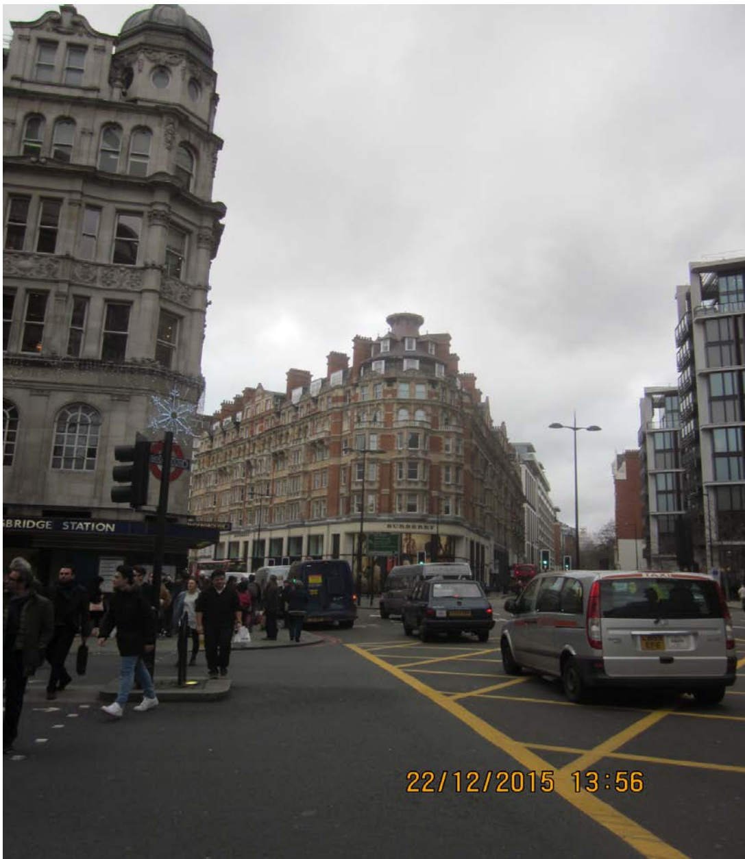
Long View from the east
